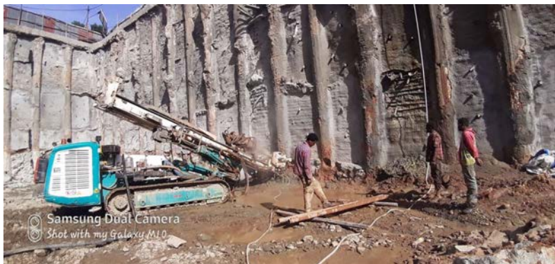
Shoring Pile Drilling and Concrete Casting of Noah Real Estate (6B+G+20 Apartment Building)
