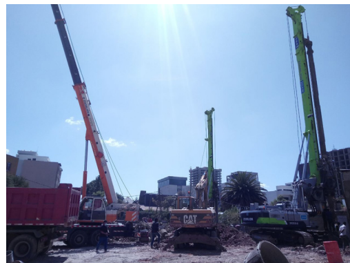
Shoring Pile Drilling and Concrete Casting of Noah Real Estate (6B+G+20 Apartment Building)
