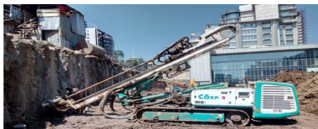
C6-XP2 ANCHOR DRILLING RIG
