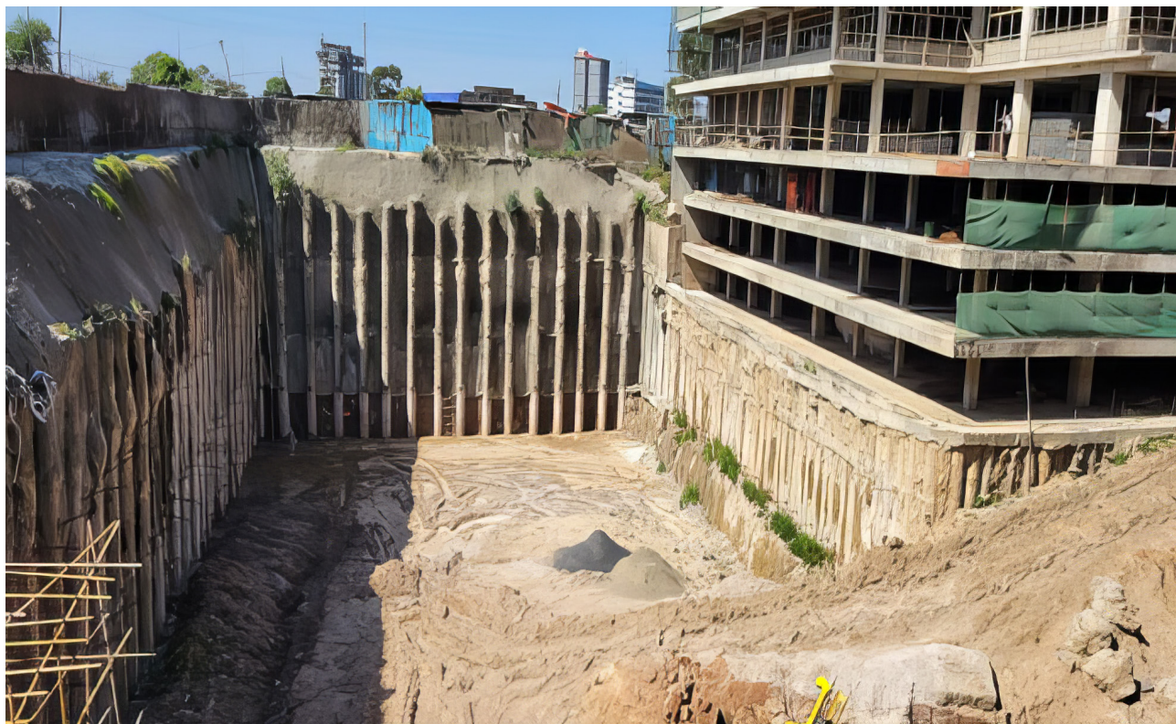
6B+G+28 Building of Yekatiit Paper Converting Plc
