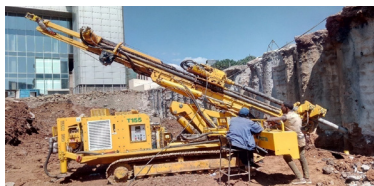
BERETTA T155 ANCHOR DRILLING RIG
